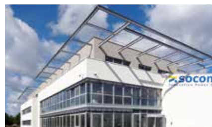
Socomec Green Building.
