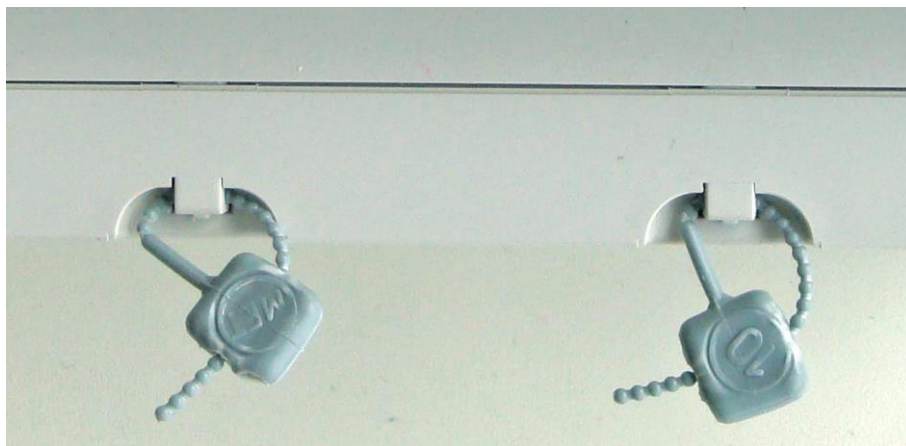
Figure 4 - Meter protection after installation
