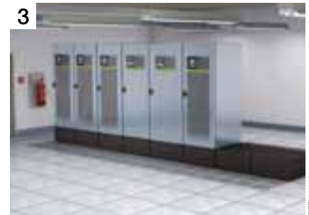
30 minutes later: 800 kW, online double conversion mode
