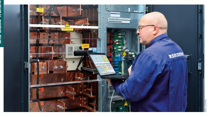
The commissioning of a UPS covers start-up of the equipment, verification of its functions according to its design specifications, and to ensure that it is compatible with the customer's working environment.
