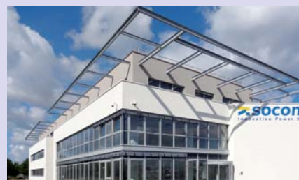
Socomec Green Building.
